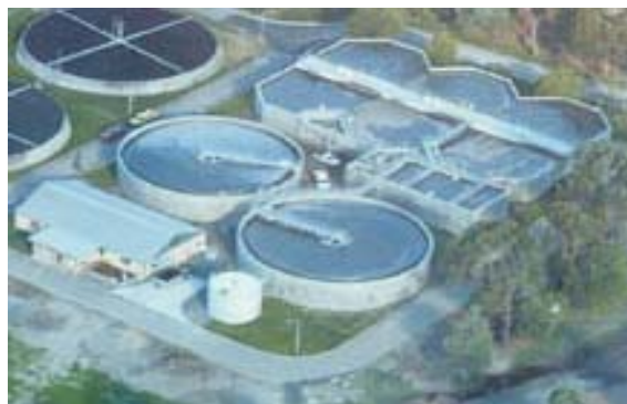
Figure 10.7 An aerial view of a sewage plant
